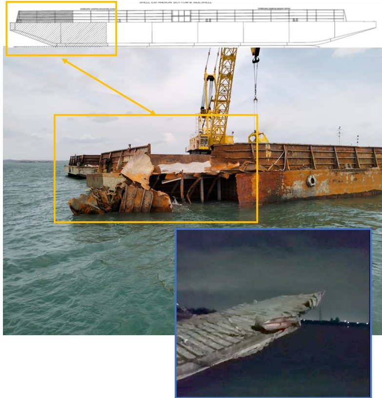
Figure 20 – Hull damage on the barge SOL2 and damage bow ramp door (inset) (Source: SOL1)
